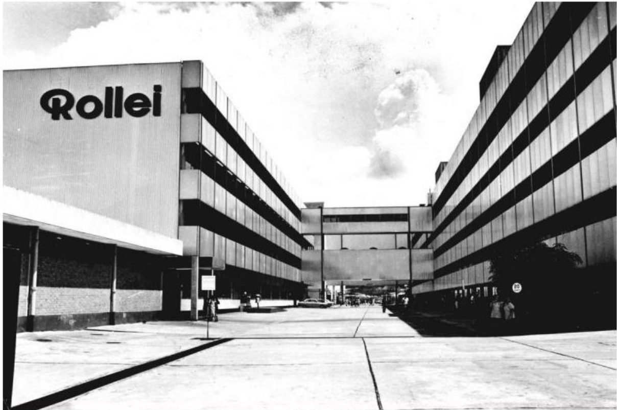
The Rollei factory in Singapore. PHOTO: ST FILE
